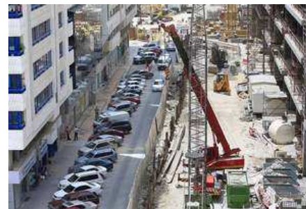
Contractors working in Abu Dhabi have to deal with a variety of codes culled from British, American and Australian standards. Ravindranath K / The National
